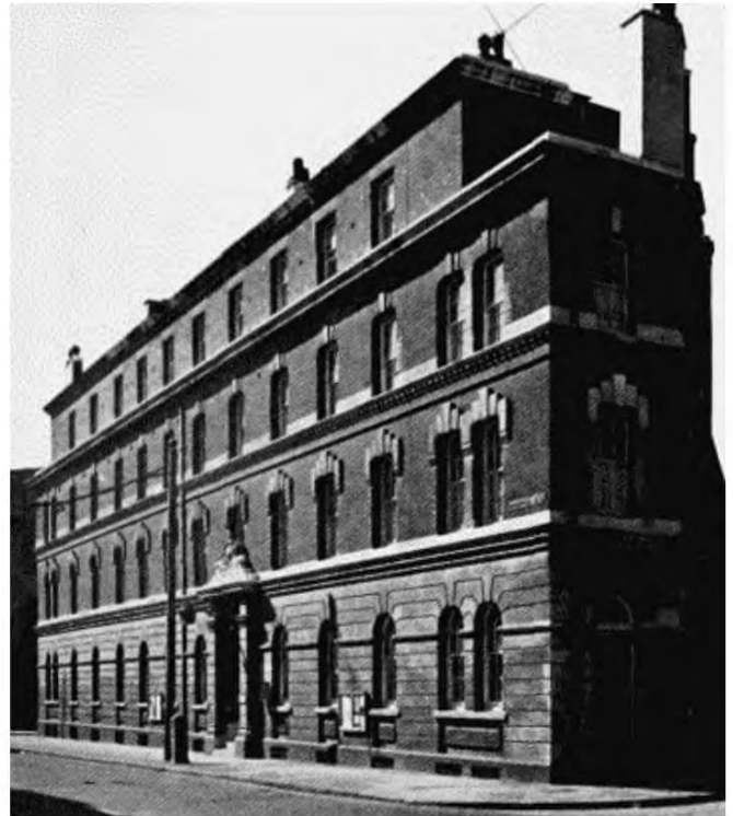
Commercial Street Police Station
